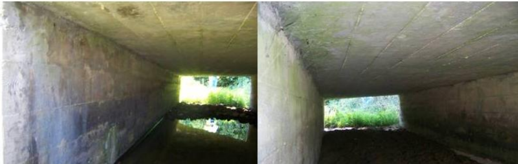
Figure 5: Inner Structure of Box Culvert
